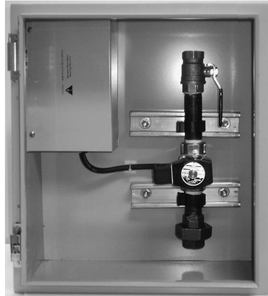
Natural Gas Solenoid Assembly Shown
